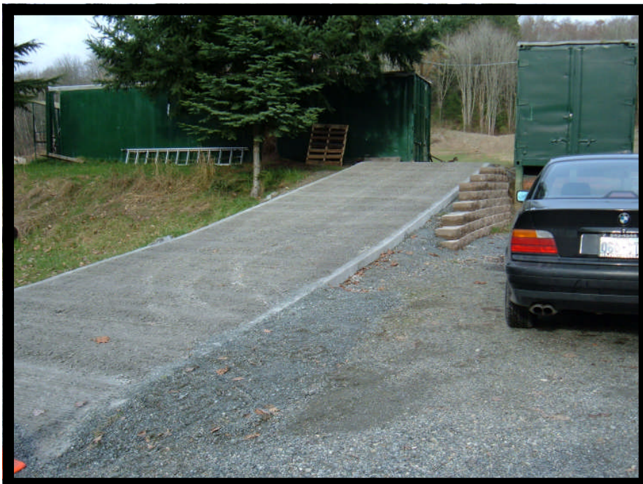
New cement equipment and supplies ramp from west parking lot.
